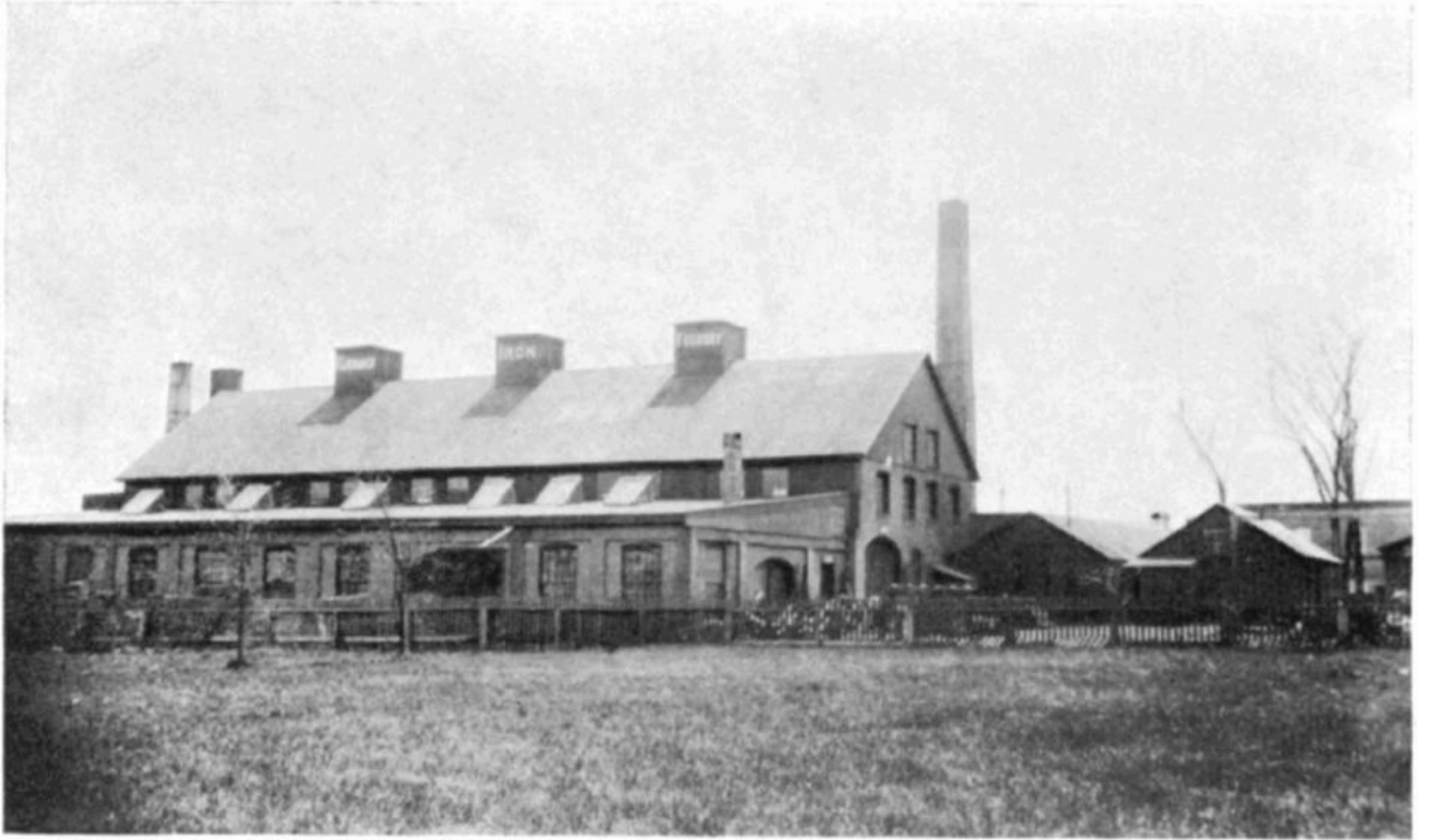
Fairhaven Iron Foundry. Erected 1843 as a Cotton Mill. Tabitha Inn, Our Lady's Haven placed near same site.
