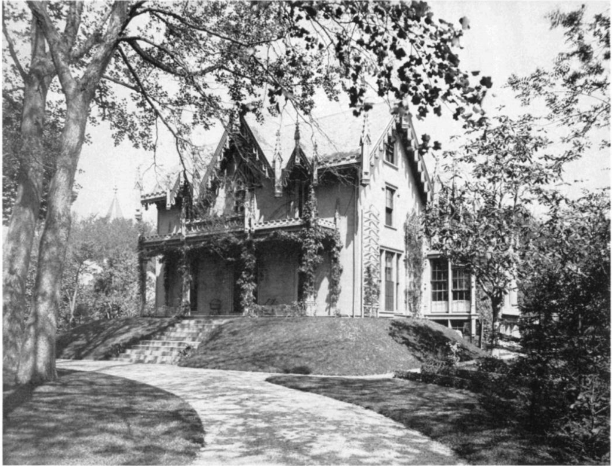
William P. Jenney House, Faced Union St., N. W. Cor. Green Street
